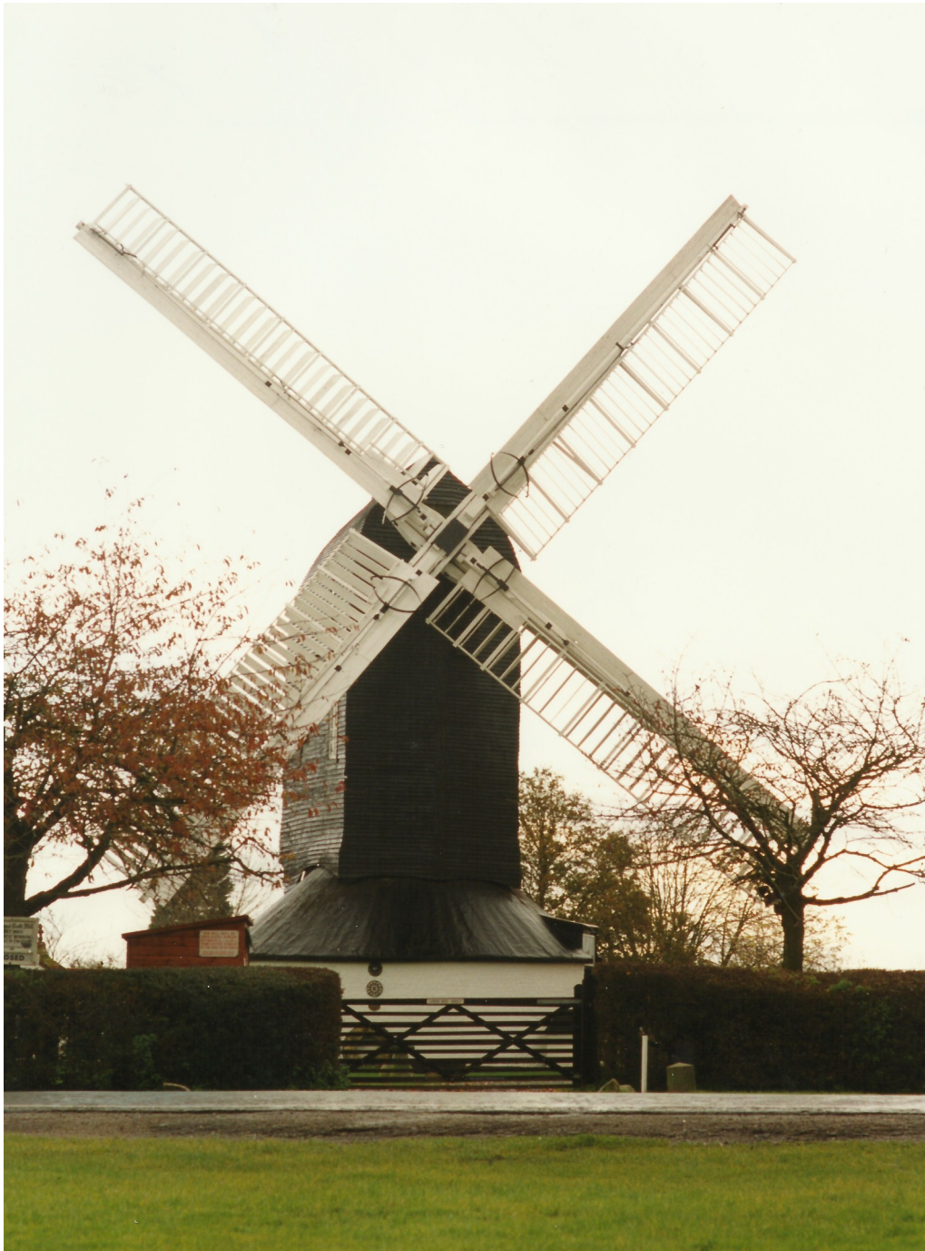
Outwood post mill.
