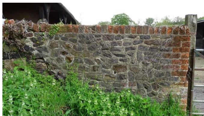
This section obviously repointed, or rebuilt more recently, with an older part to the left.
