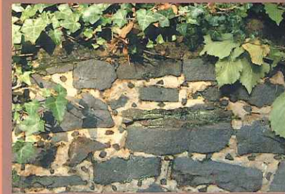
Ironstone has been used to build this wall in Albury, with smaller fragments decorating the mortar.
