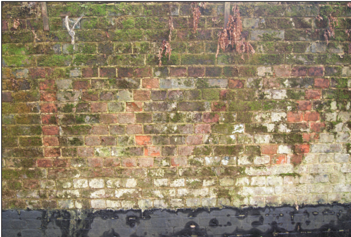
Plate 13: Date '1873' built into brickwork of expense magazine
